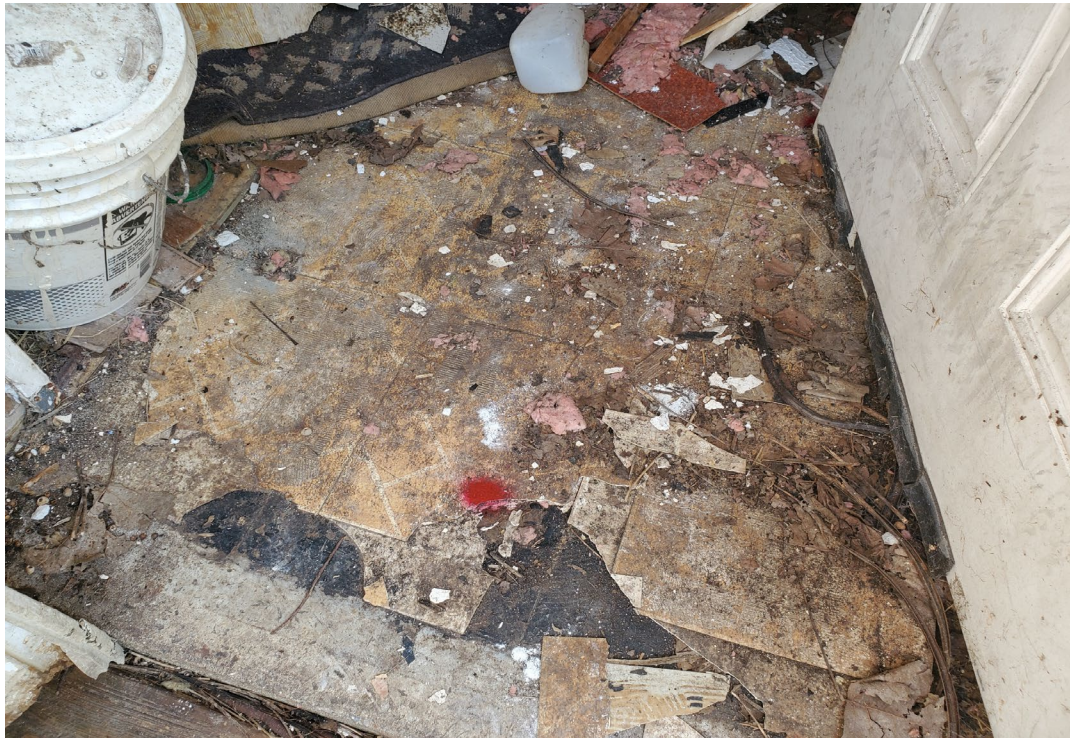
PHOTO: 4 BY: A. Paquet SUBJECT: Rear Entry Floor Tile Multilayer with Mastic
