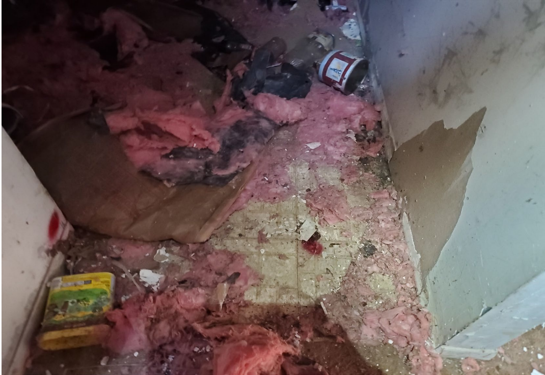
PHOTO: 3 Kitchen 12"12" Tan Floor Tile Multilayer/Mastic BY: A. Paquet SUBJECT:
