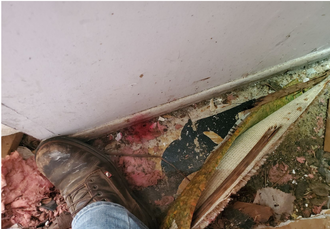
PHOTO: 2 SUBJECT: Living 12"x12" Floor Tile with Mastic
