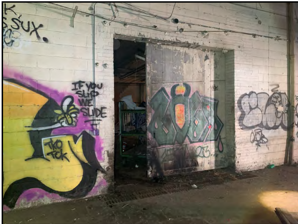
Photo 8: View of the trench drain located between the eastern and central areas of the subject property building.
