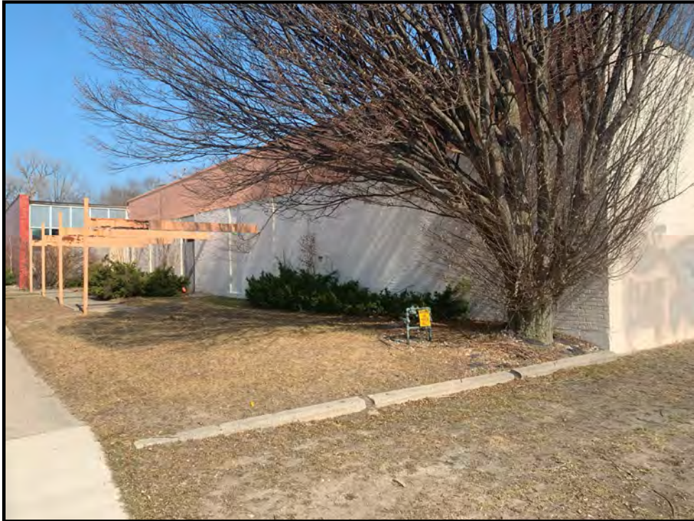
Photo 1: View to northeast from the southwest corner of the subject property.
