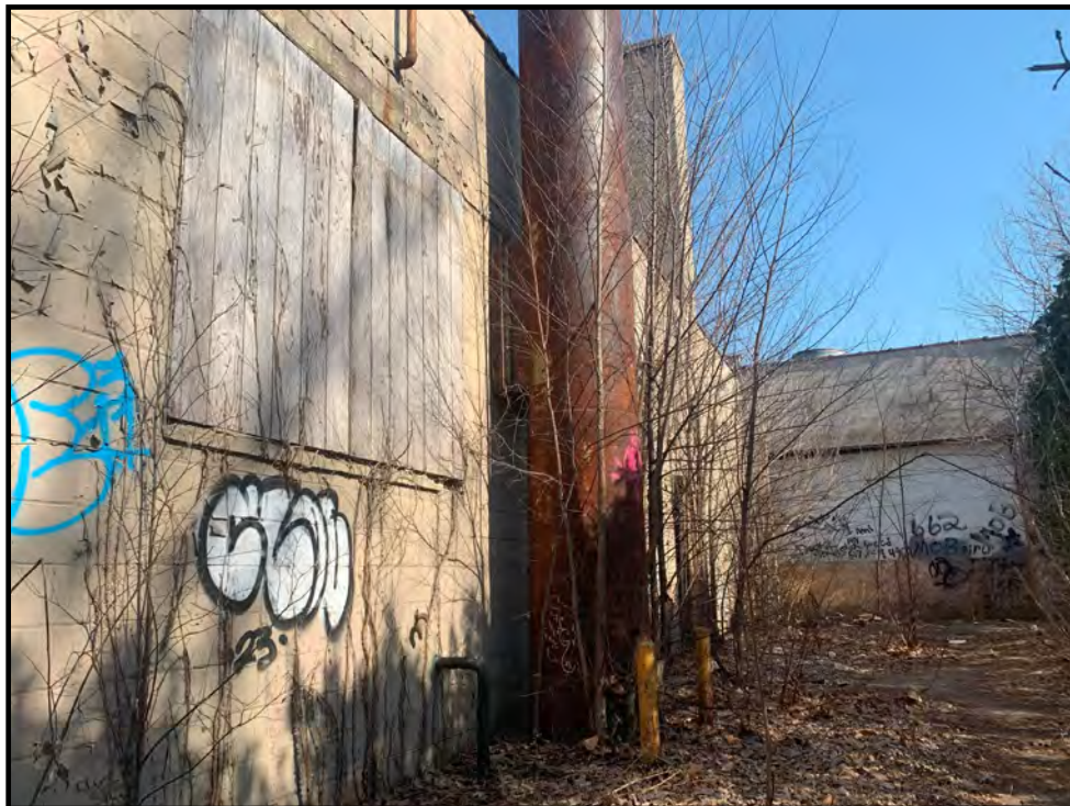
Photo 16: View of the former location of the removed 10,000-gallon gasoline UST, located south of the central portion of the subject property building.
