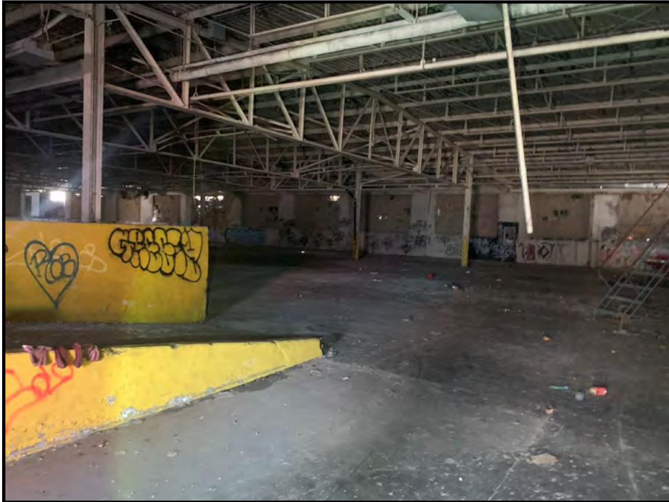
Photo 5: View of the northeastern portion of the warehouse within the subject property building.
