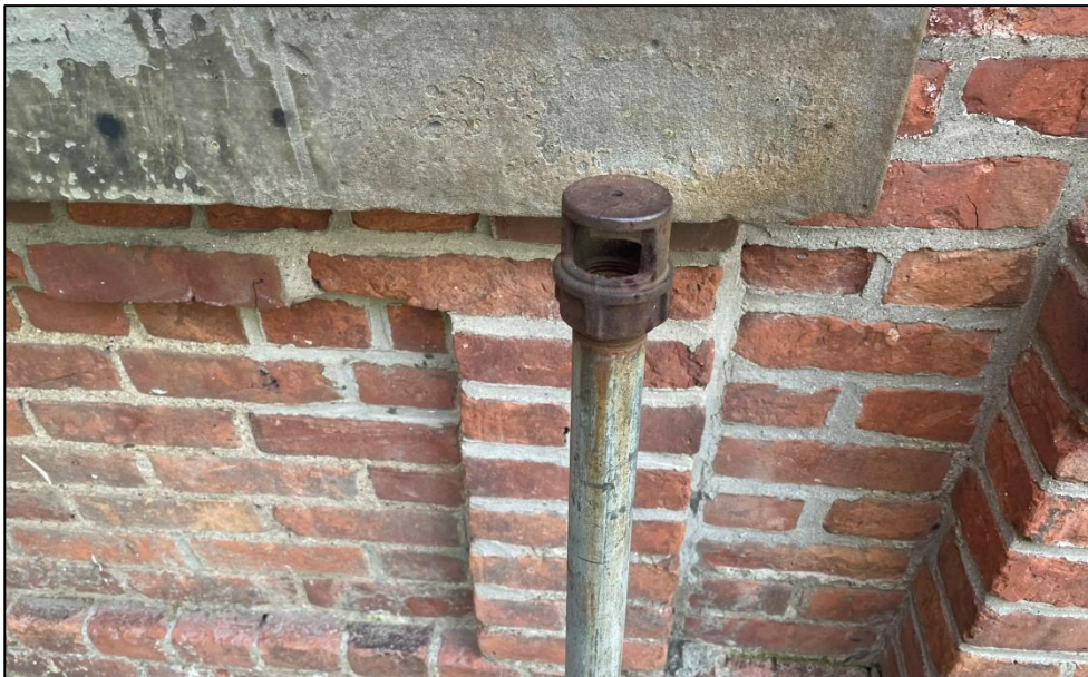
Photo 8: View of a suspect heating oil vent pipe located proximate the northwest portion of the subject property building.
