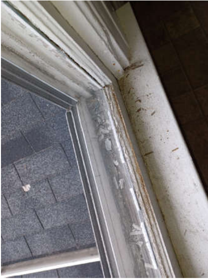
Assumed Positive: Wood Window Trough- Wells & Jambs
