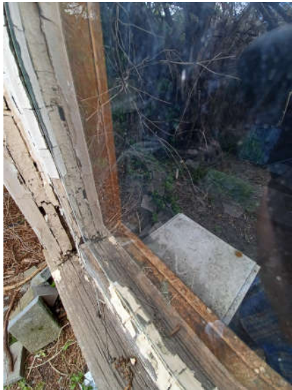
Garage Interior 19 Side B
