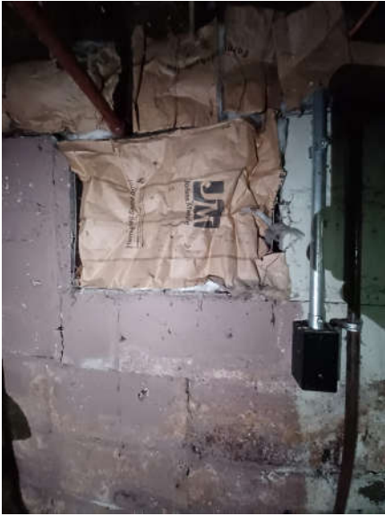
Utility Room 18 Coal Door
