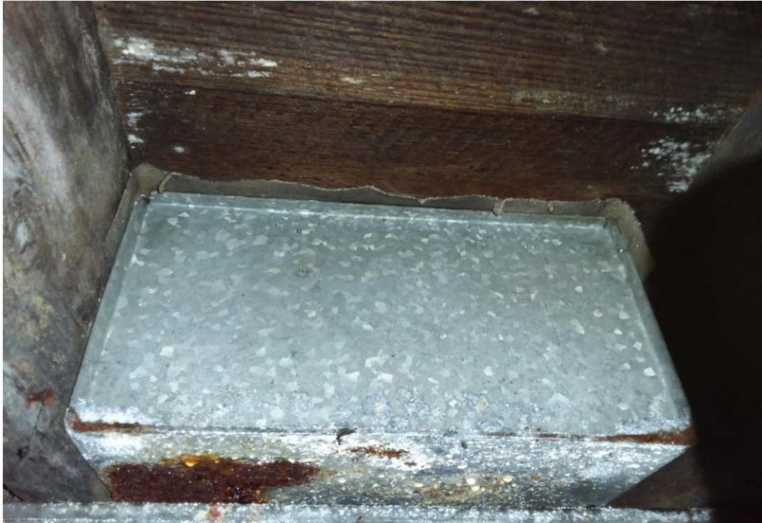
PHOTO: 3 SUBJECT: Typical HVAC Duct Boot Wrap
