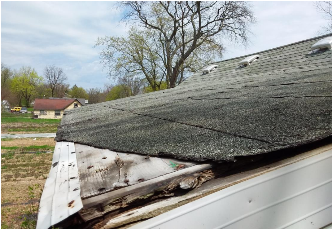
PHOTO: 2 SUBJECT: View of ACM Roofing/Tar (2nd Fl. W Dormer)
