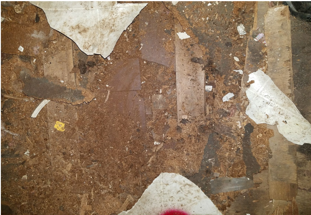
PHOTO: 2 SUBJECT: Kitchen Brown 9x9 Tile beneath Raised Floor System
