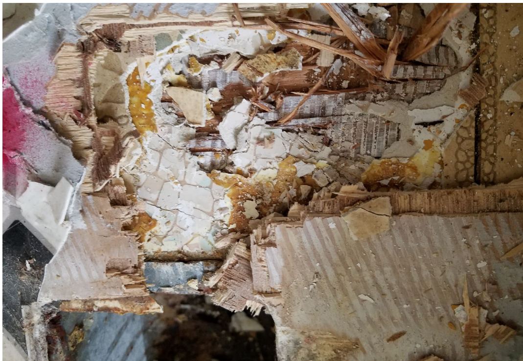
PHOTO: 2 SUBJECT: Asbestos Flooring in W Bathroom
