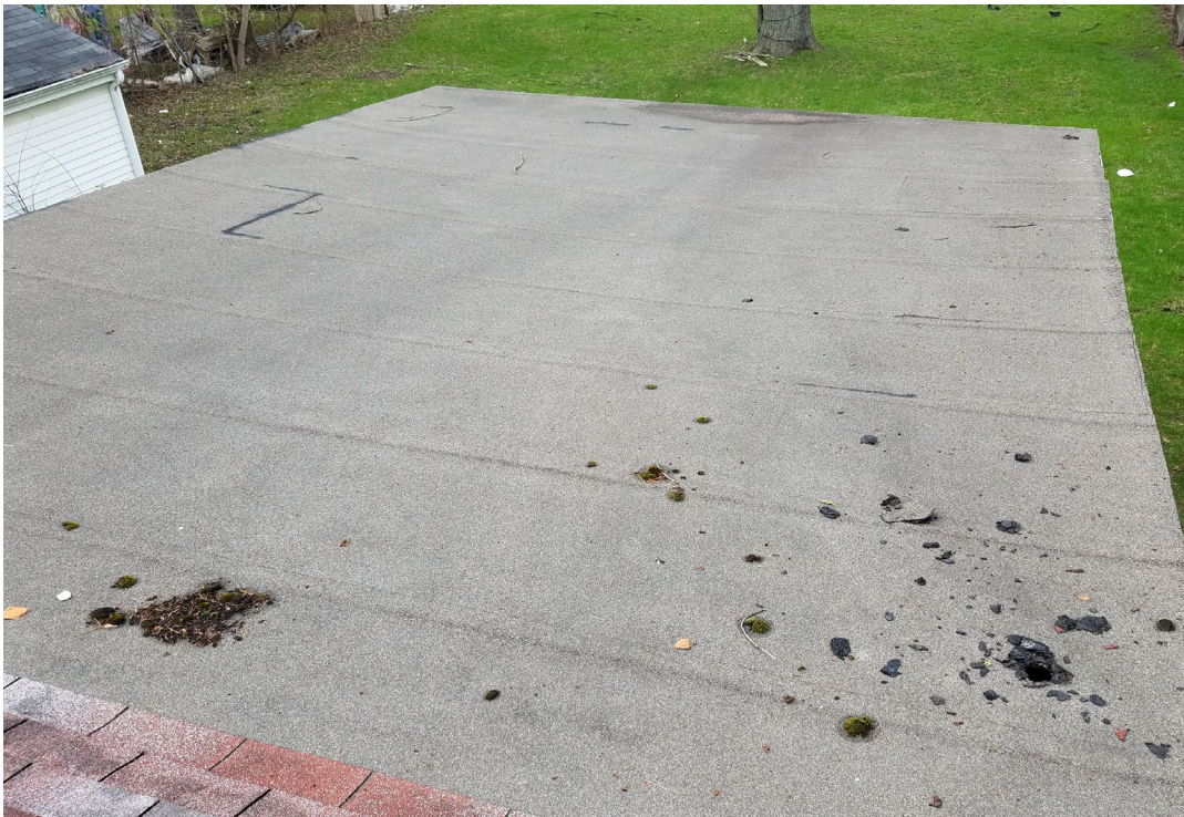
PHOTO: 6 SUBJECT: Asbestos Roofing (bottom layer is asbestos) on Rear Entry
