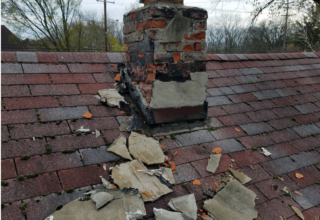
PHOTO: 5 SUBJECT: Asbestos Chimney Flashing
