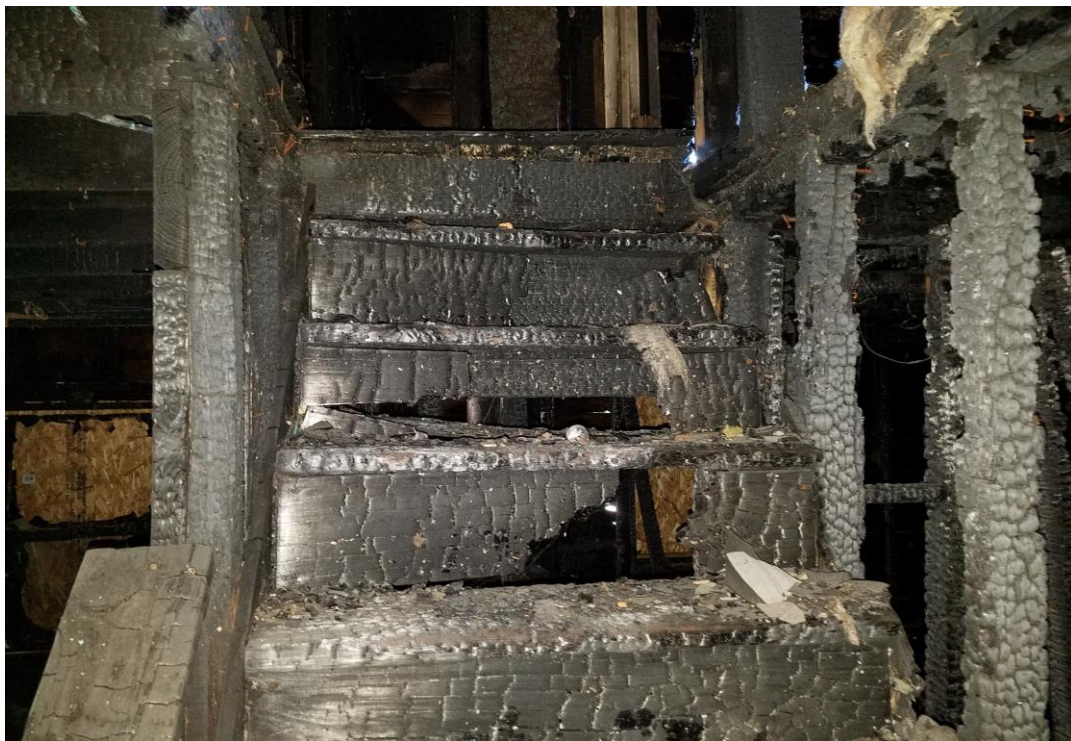
PHOTO: 2 SUBJECT: Fire Damaged Stairwell
