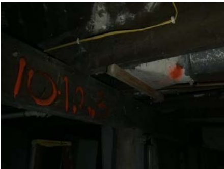
Sample ID: AS 10-1 Location: Basement Notes: Vent Wrap
