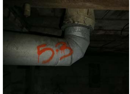
Sample ID: AS 5-3 Location: Basement Notes: Vent Wrap
