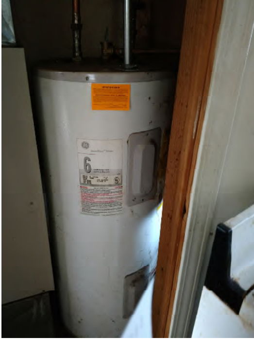
Hot Water Tank
