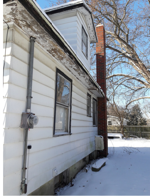
Side #1 of house/property
