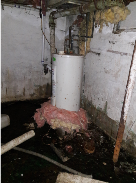
Hot Water Heater
