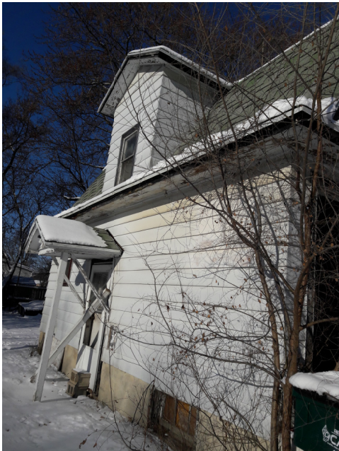
Back of house/property
