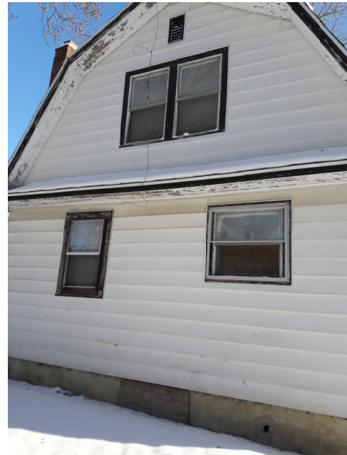
Side #2 of house/property
