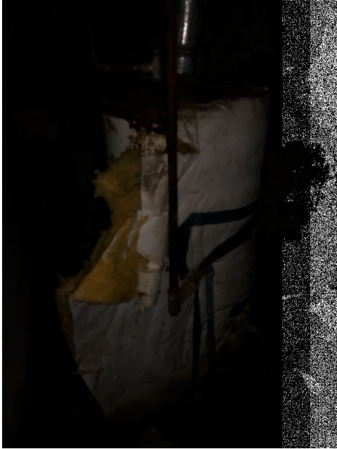
Hot Water Tank
