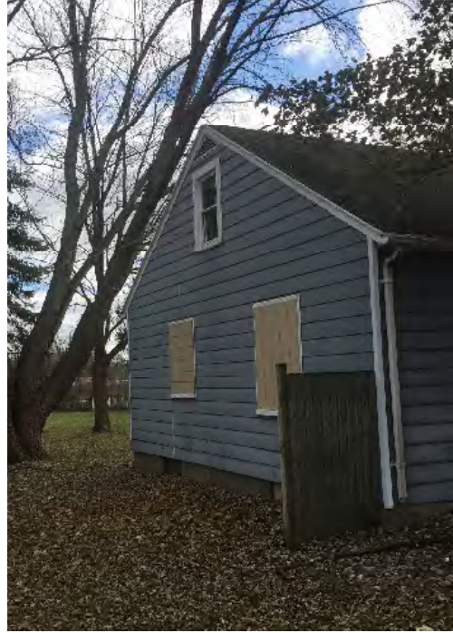
Side #1 of house/property
