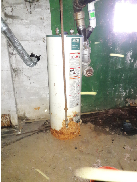
Hot Water Tank
