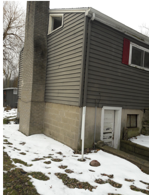
Side #1 of house/property
