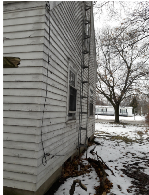
Side #2 of house/property
