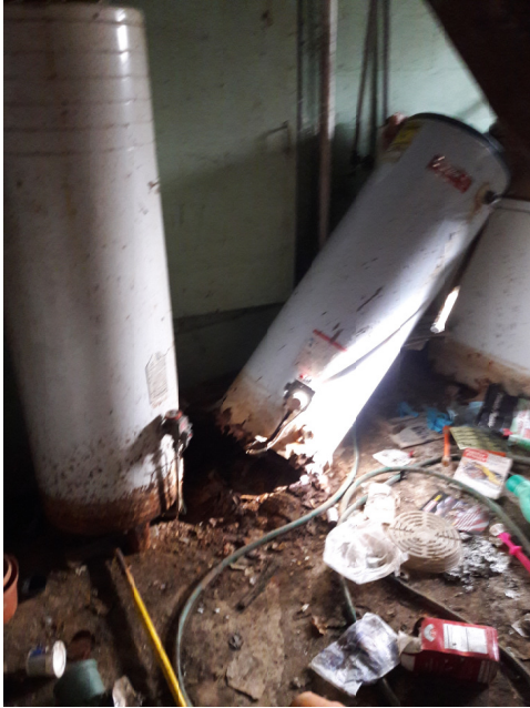
Hot Water Heater
