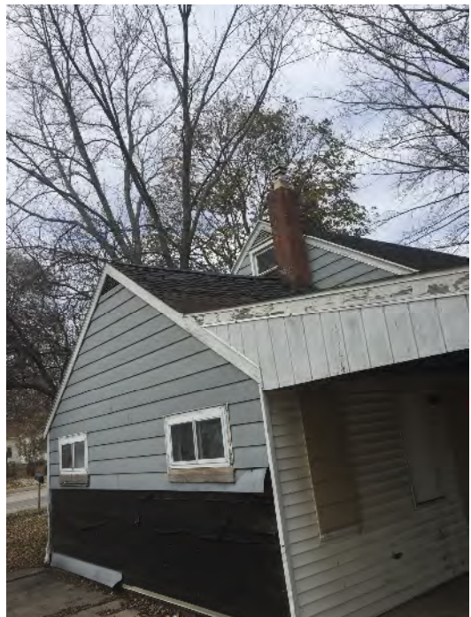
Side #2 of house/property
