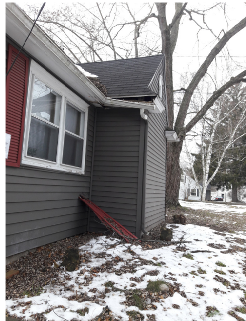
Side #2 of house/property
