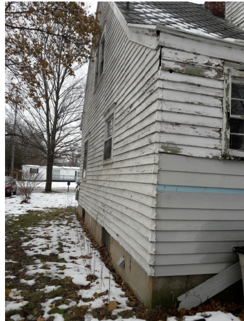
Side #1 of house/property
