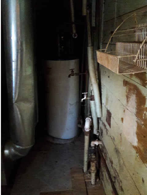
Hot Water Tank
