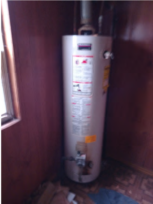
Hot Water Heater
