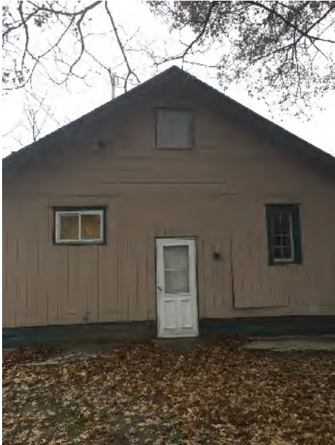
Back of house/property
