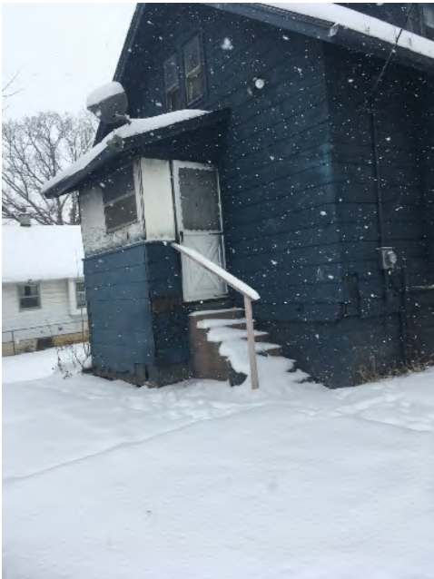
Back of house/property
