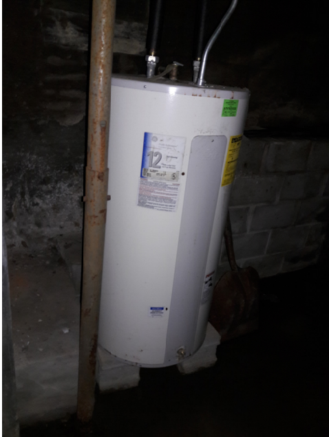
Hot Water Tank
