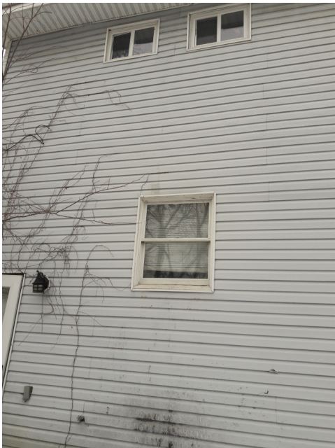
Back of house/property
