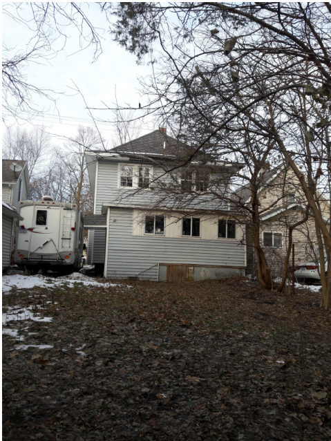
Back of house/property
