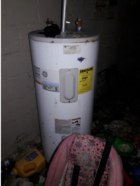
Hot Water Heater
