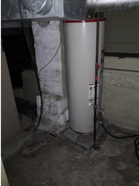
Hot Water Heater
