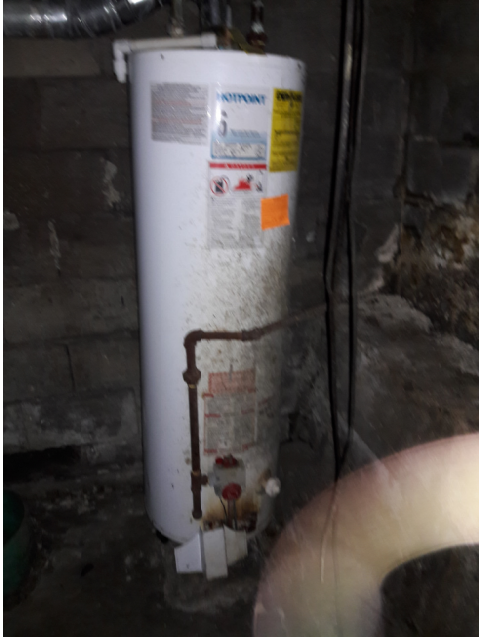
Hot Water Tank
