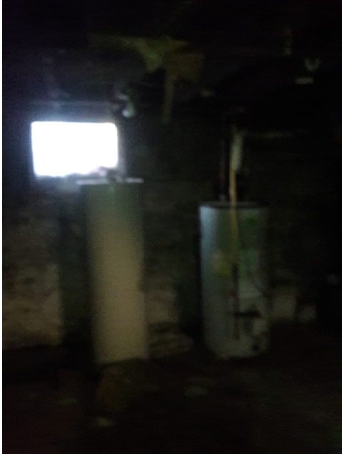
Hot Water Heater
