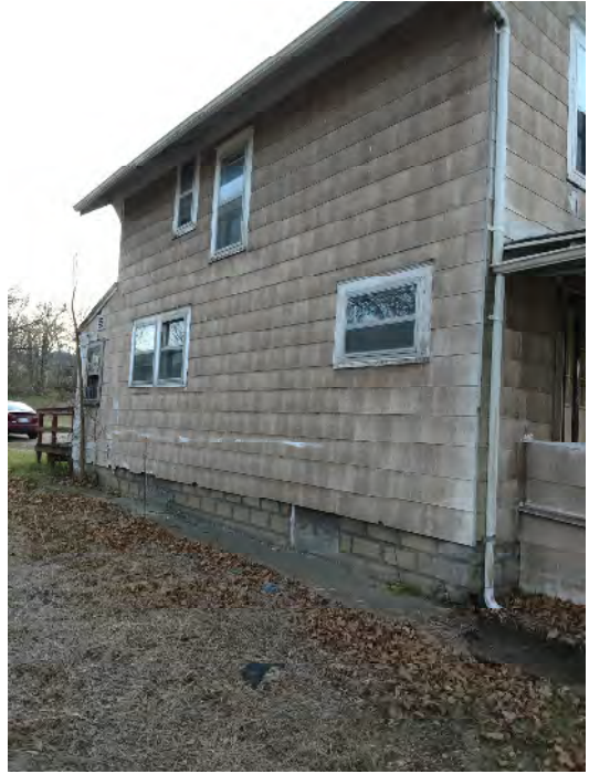
Side #1 of house/property
