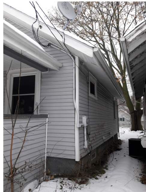
Side #2 of house/property
