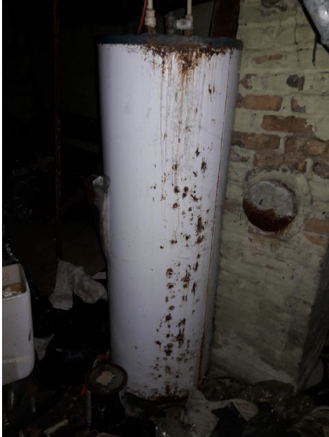
Hot Water Heater
