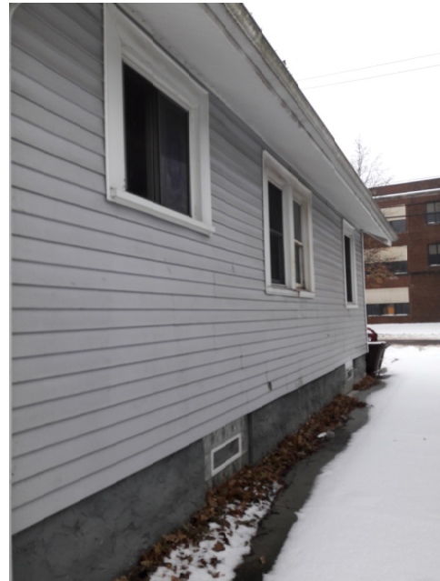
Side #1 of house/property
