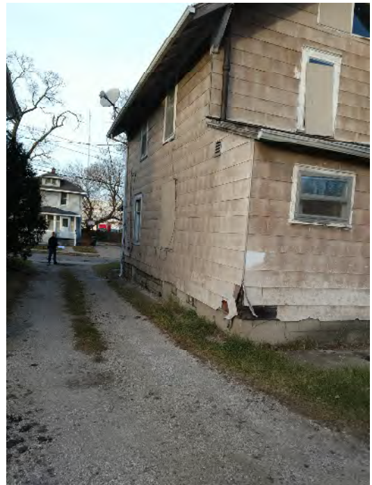
Side #2 of house/property
