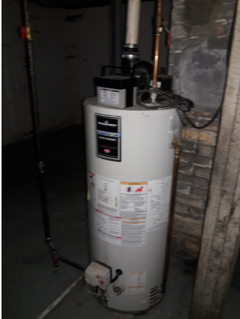
Hot Water Tank
