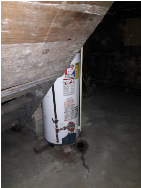
Hot Water Tank
