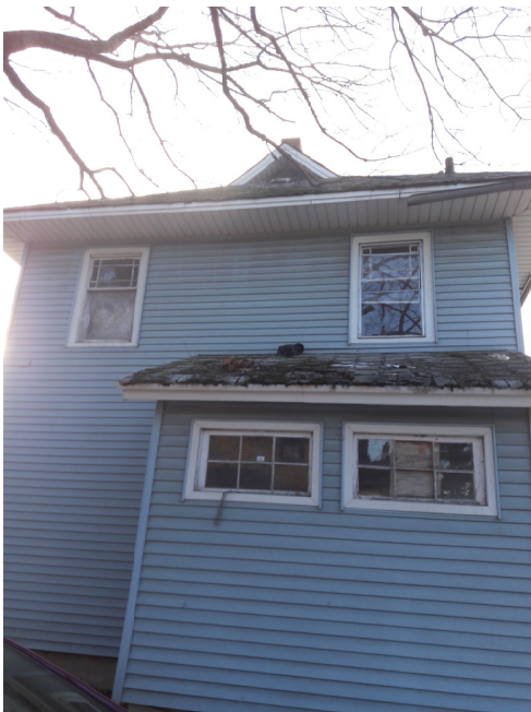
Back of house/property
