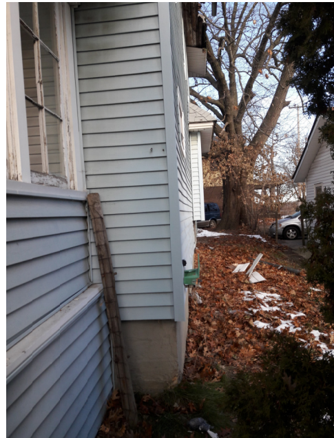
Side #2 of house/property
