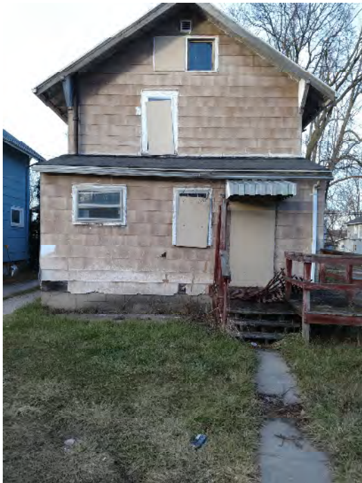
Back of house/property
