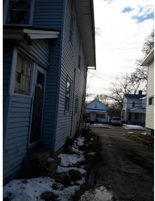
Side #1 of house/property
