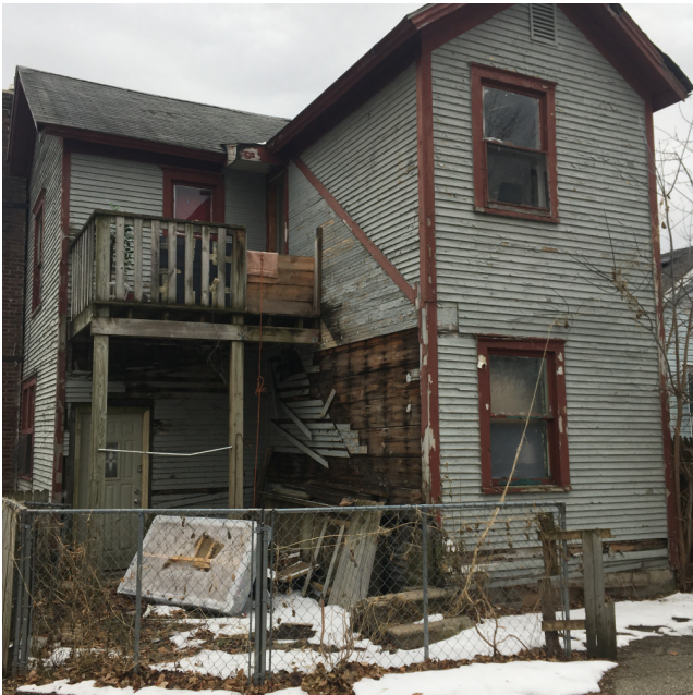
Back of house/property
