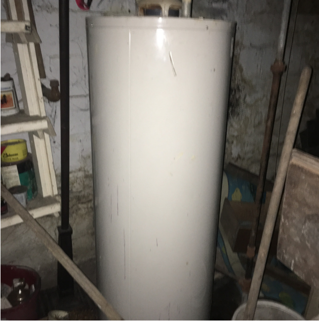
Hot Water Tank
