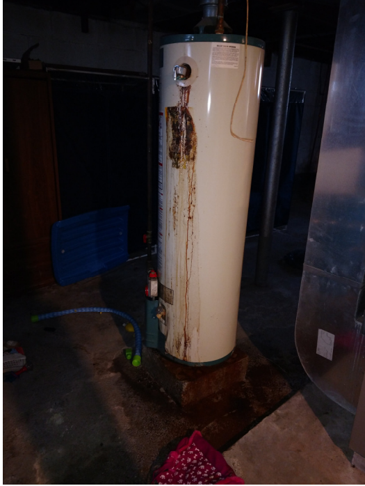
Hot Water Tank
