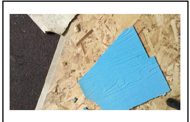
Siding sample from exterior second story
