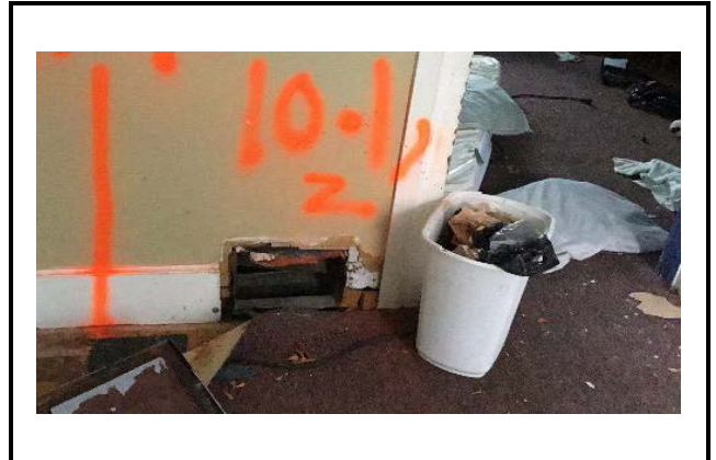
Vent wrap sample from room 8
