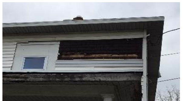
Asphalt siding sample from exterior
