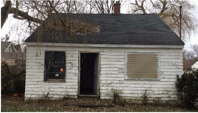
1311 N MLK Jr Blvd, Front of House
