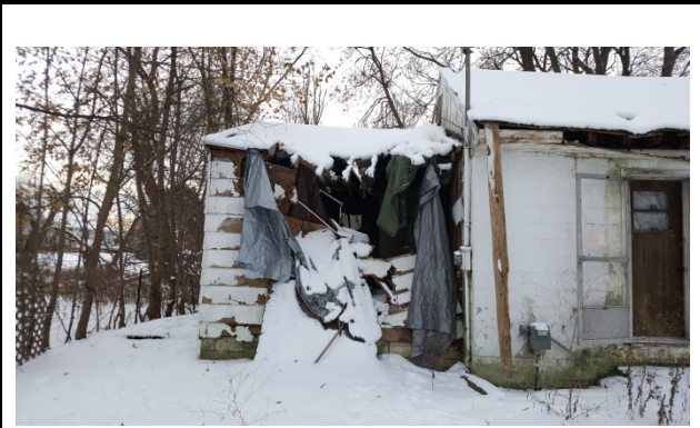
View of collapsed eastern portion of house
