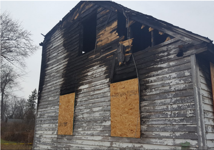
South side of house.
