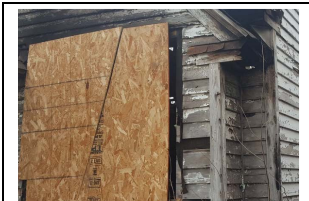
Exterior siding tar paper sample AS2-1
