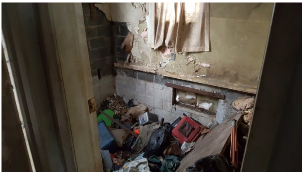
Collapsed floor in southwestern portion of house
