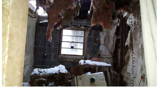
View of southeastern portion of house
