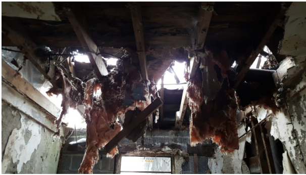
Collapsed ceiling in southeastern portion of house
