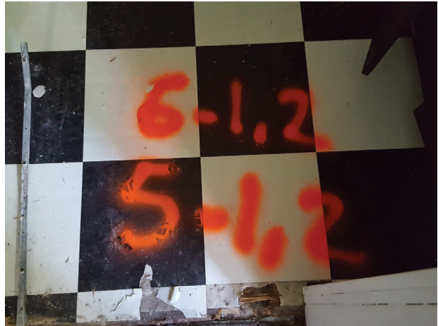
Two Flooring Layers in Room 4
