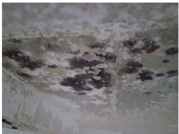
Drywall Ceiling with Mold in Basement
