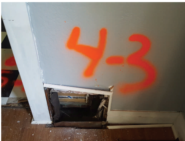
Room 3 Vent with Vent Wrap
