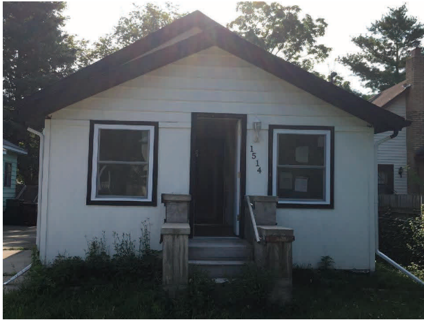
1514 Illinois Ave. Front of House
