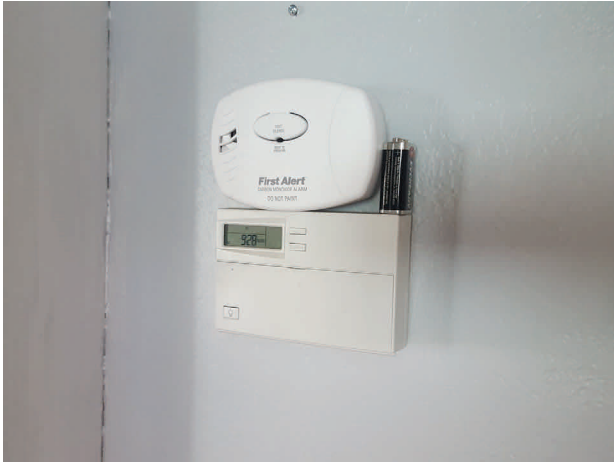
Electric Thermostat and Carbon Monoxide Detector in Hall
