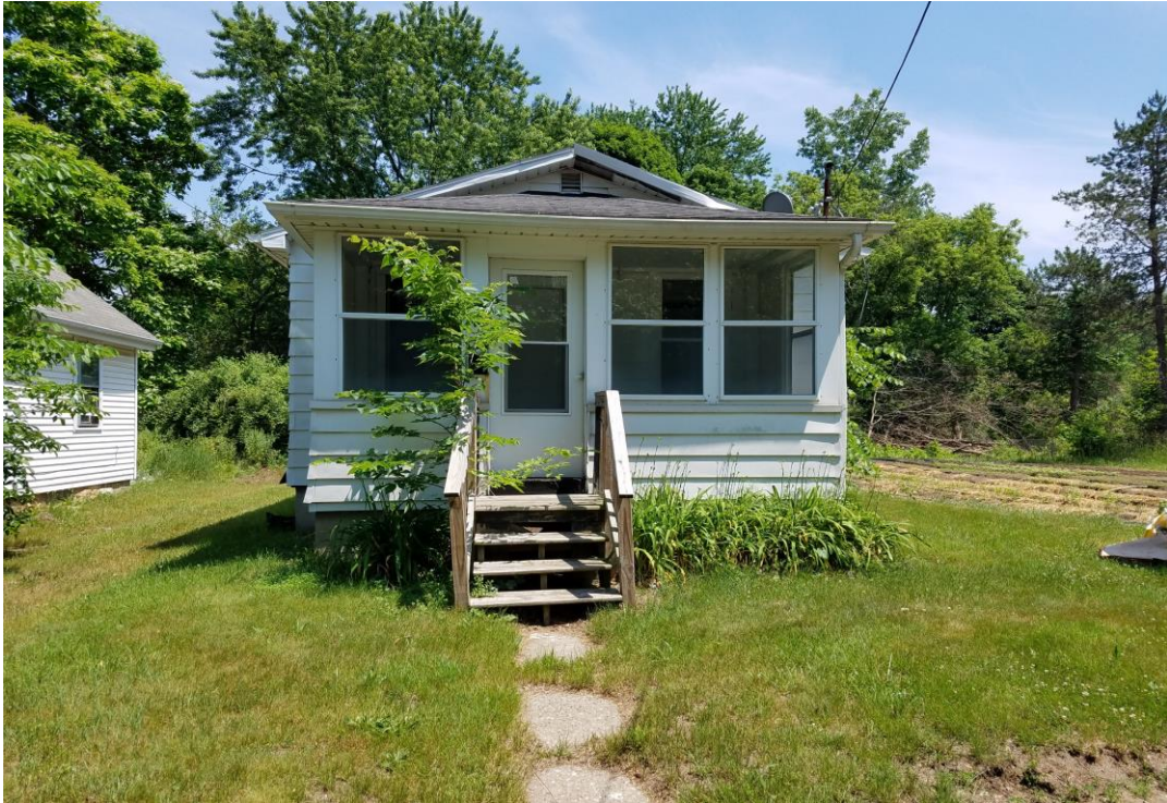
PHOTO: 1 SUBJECT: View of front of the Property.
