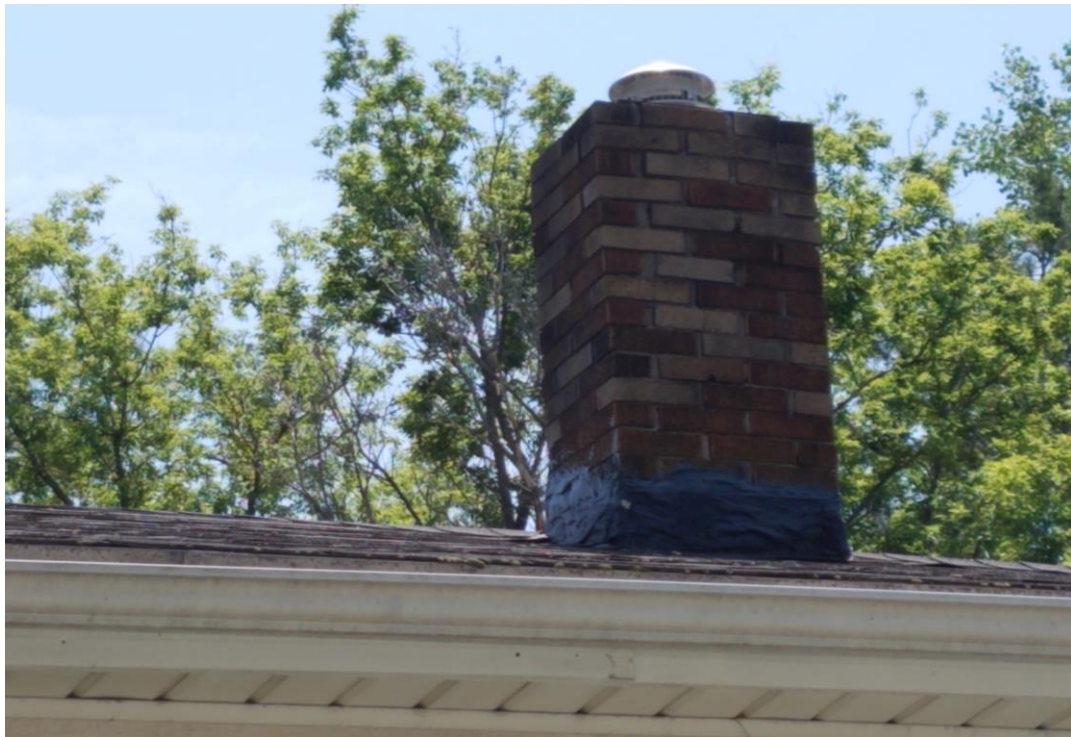
PHOTO: 2 SUBJECT: Chimey Flashing
