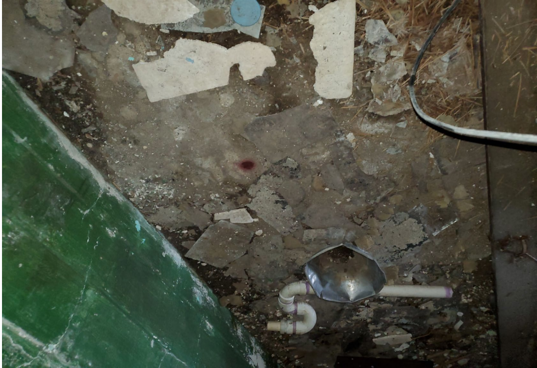
PHOTO: 3 Basement and Stairwell Brown 9x9 Tile SUBJECT:
