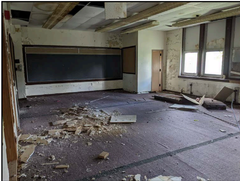
Photo 6: View of a former classroom within the subject property building.
